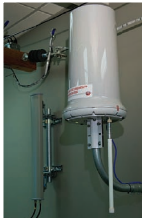
WiMax, 3G Cellular, Trilliant, and Silver Spring WAN and FAN Access Points
